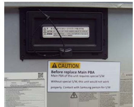
Example of label on outdoor unit
